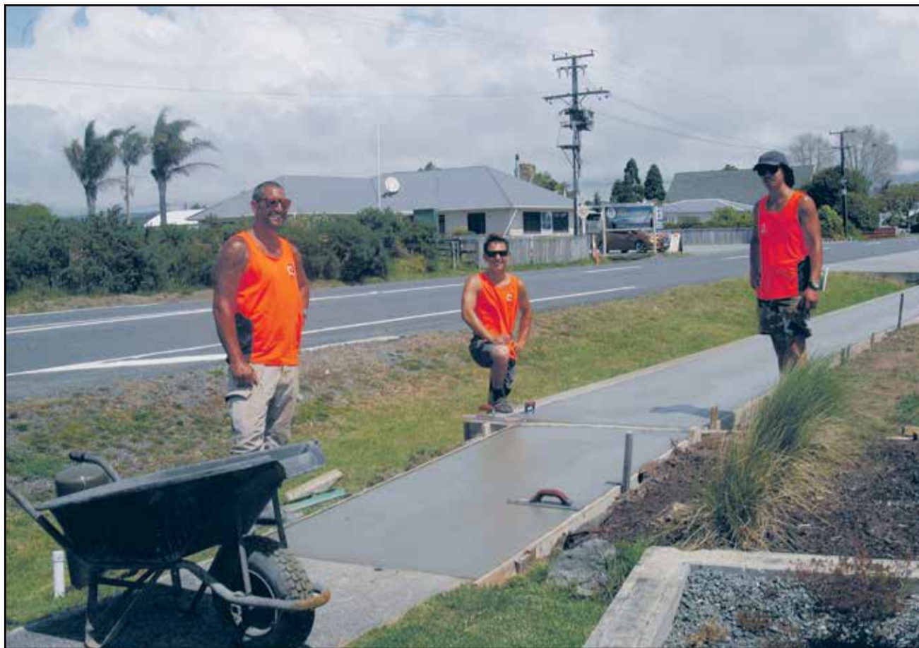
The team from Complete Concrete laying the new footpath:from left: Dion Webb, Shaun Davis and Paul Dey
